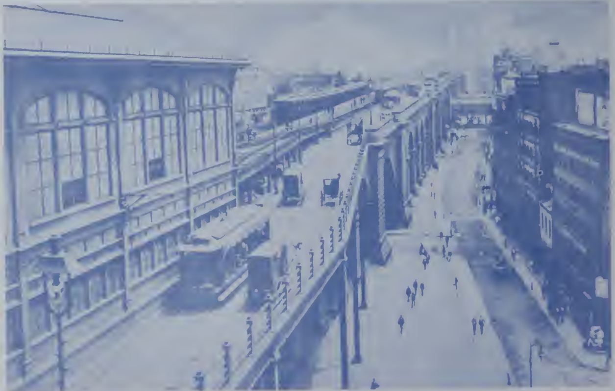
The bridge approach from Manhattan in 1899, showing wagon road, trolley line, elevated cars and promenade
